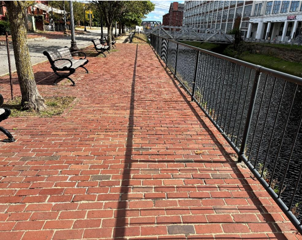
Photo 17 – Walkway Along North Canal
