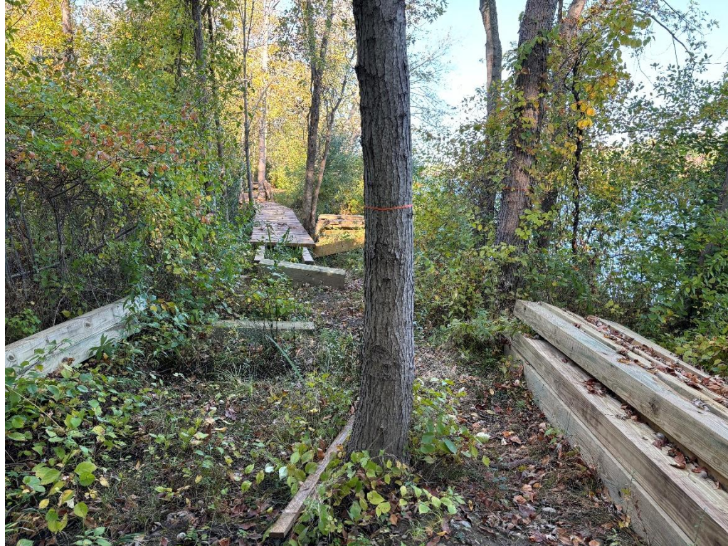
Photo 3 Trail Maintenance and Construction
