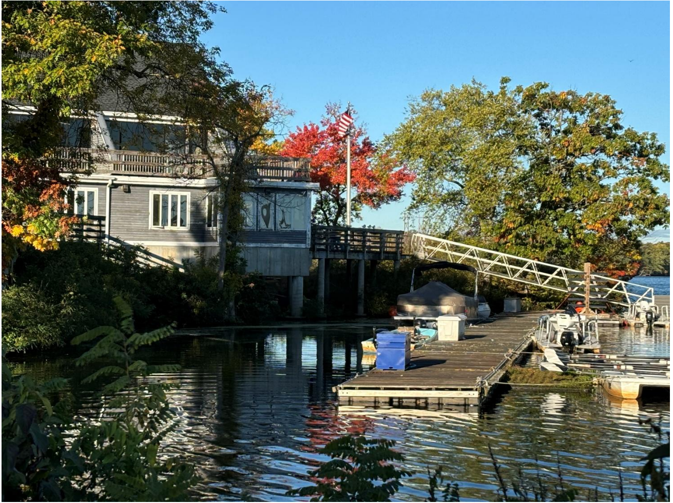
Photo 15 – Ramp and Floating Dock
