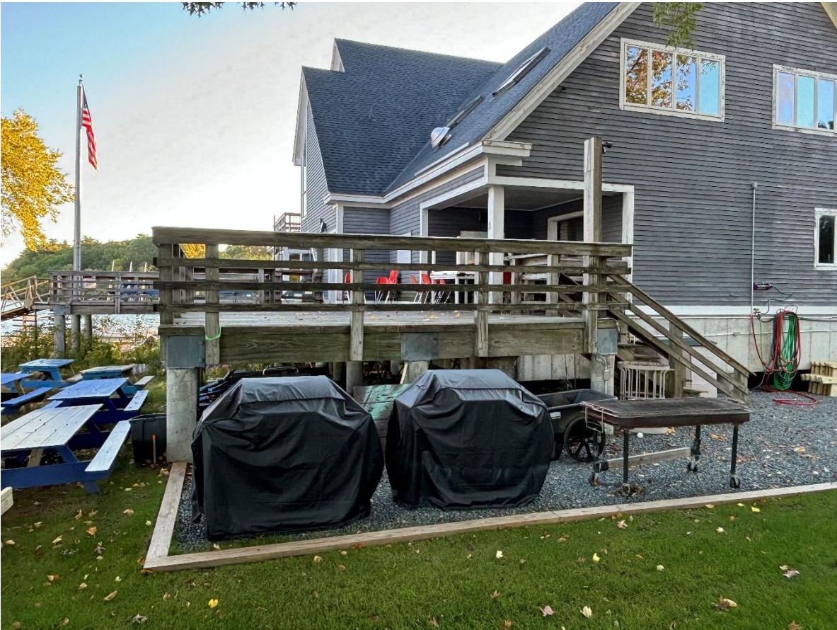
Photo 13 – Grills and Deck
