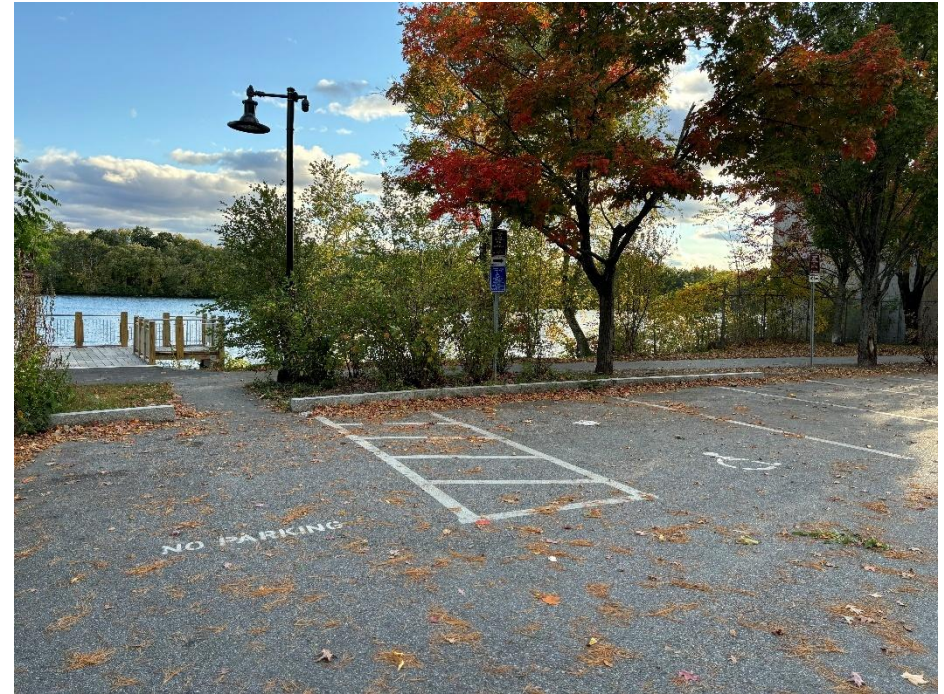
Photo 78 ADA Parking at Fishing Pier
