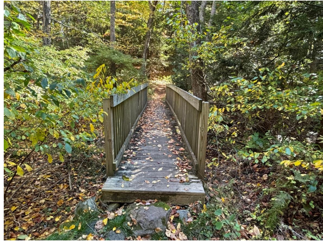
Photo 12 – Footbridge with Handrailing
