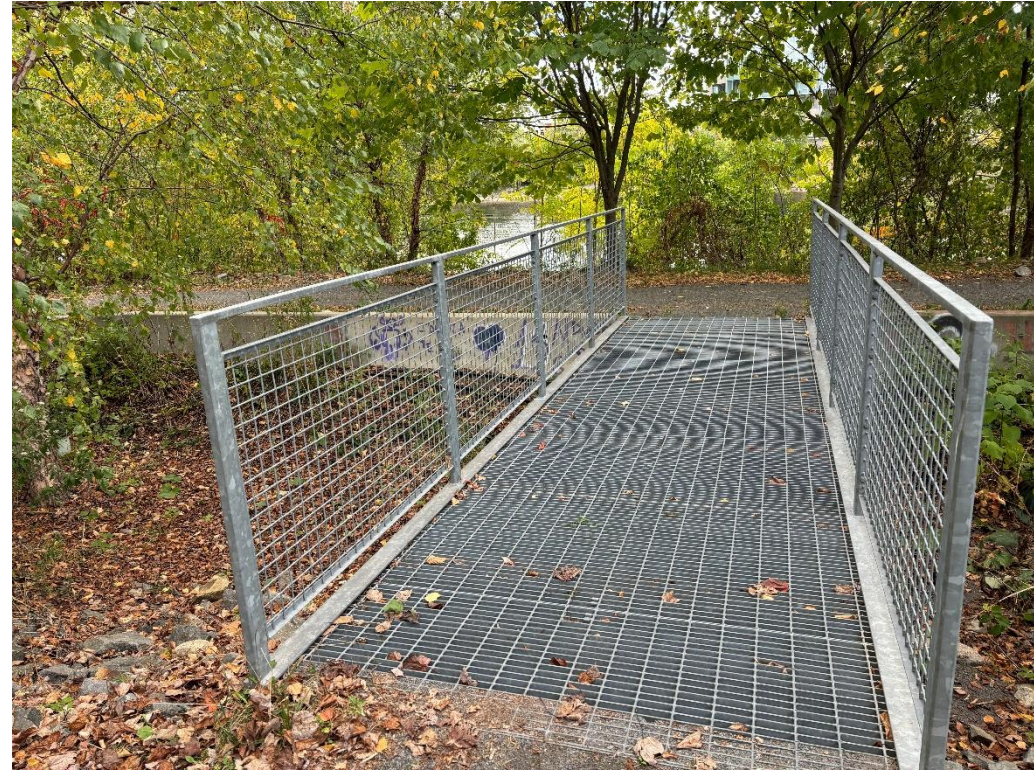
Photo 46 Pedestrian Bridge and trail
