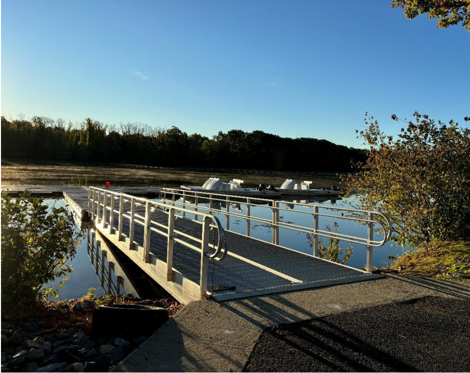
Photo 84 Dock and access ramp
