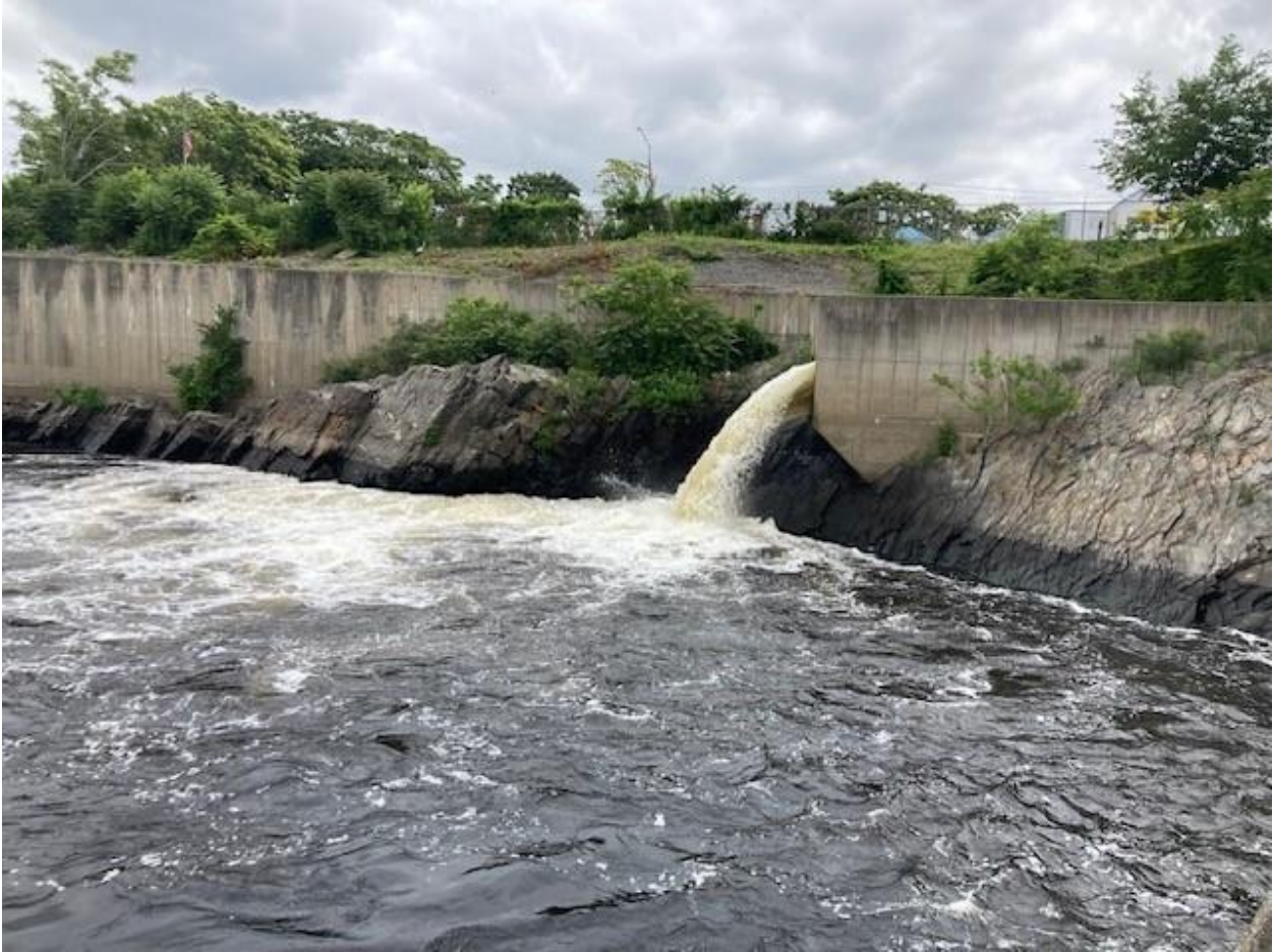
Figure 5: Water mark on ledges shows a drop of 3 – 4 feet following turbine outage for maintenance.
