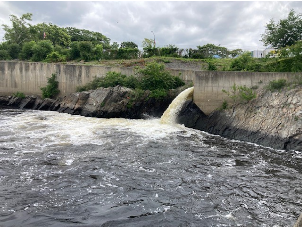
Figure 5: Water mark on ledges shows a drop of 3 – 4 feet following turbine outage for maintenance.
