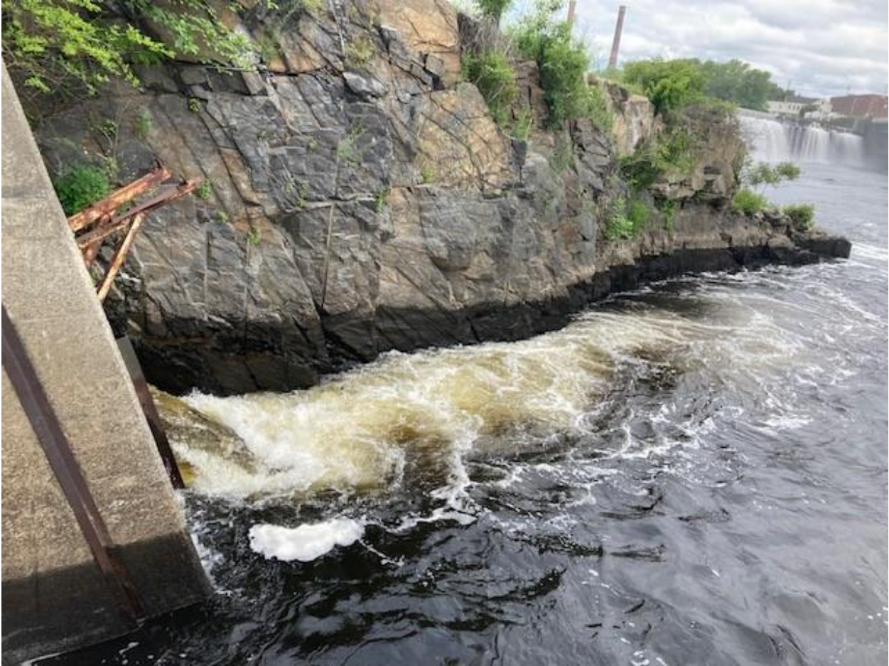
Figure 6: Perched fishway entrance conditions as water levels dropped suddenly in the tailrace.
