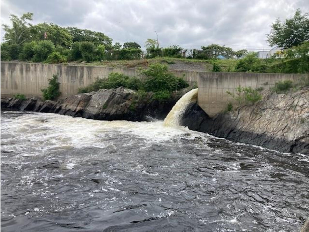
Figure 5: Water mark on ledges shows a drop of 3 – 4 feet following turbine outage for maintenance.
