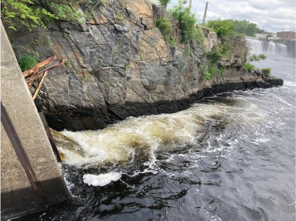
Figure 6: Perched fishway entrance conditions as water levels dropped suddenly in the tailrace.
